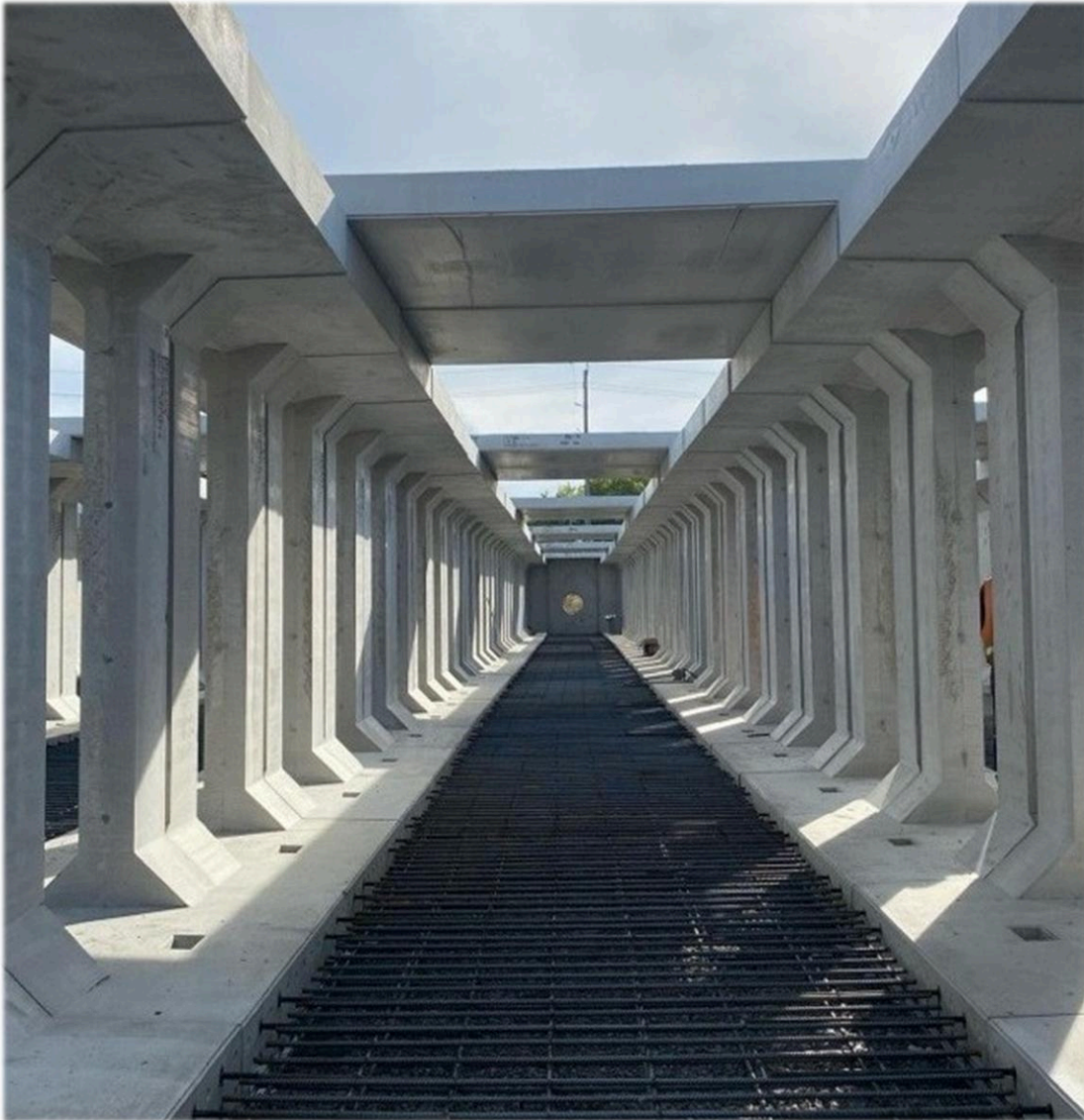
Figure 22: Cast-in-place floor reinforcement
