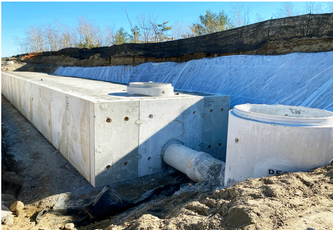
Figure 27: Fully grouted pockets and gaps
