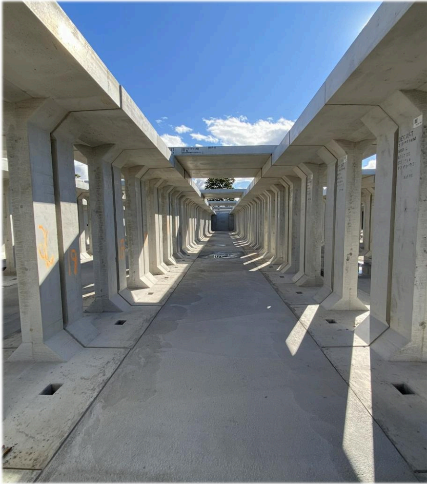
Figure 26: Finished concrete floor
