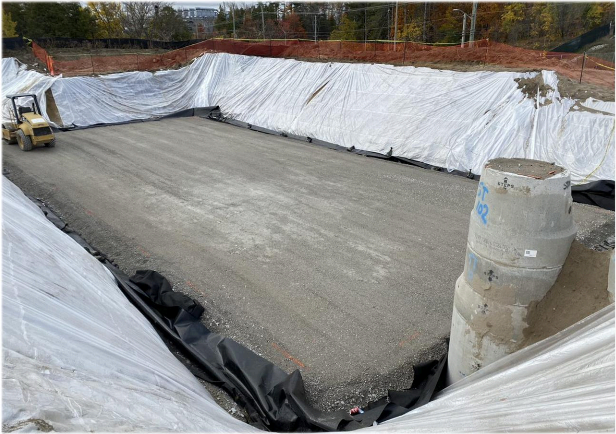
Figure 5: Example tank bedding with liner
