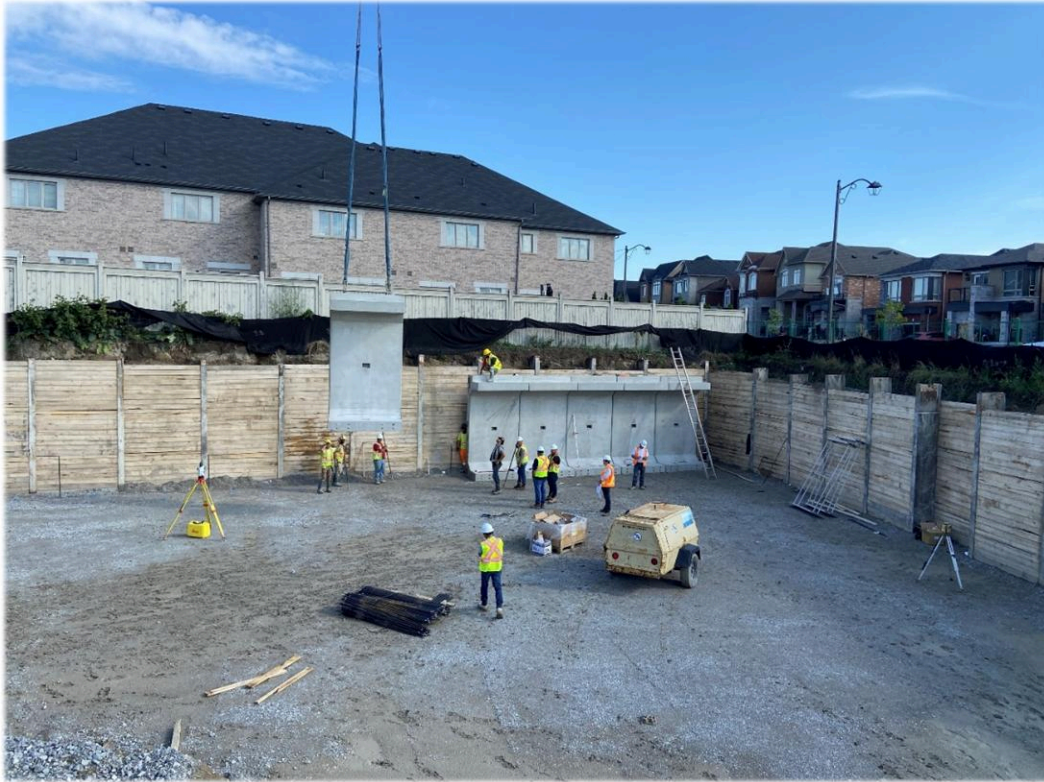
Figure 6: Installation Sequence 1 - Begin with end units
