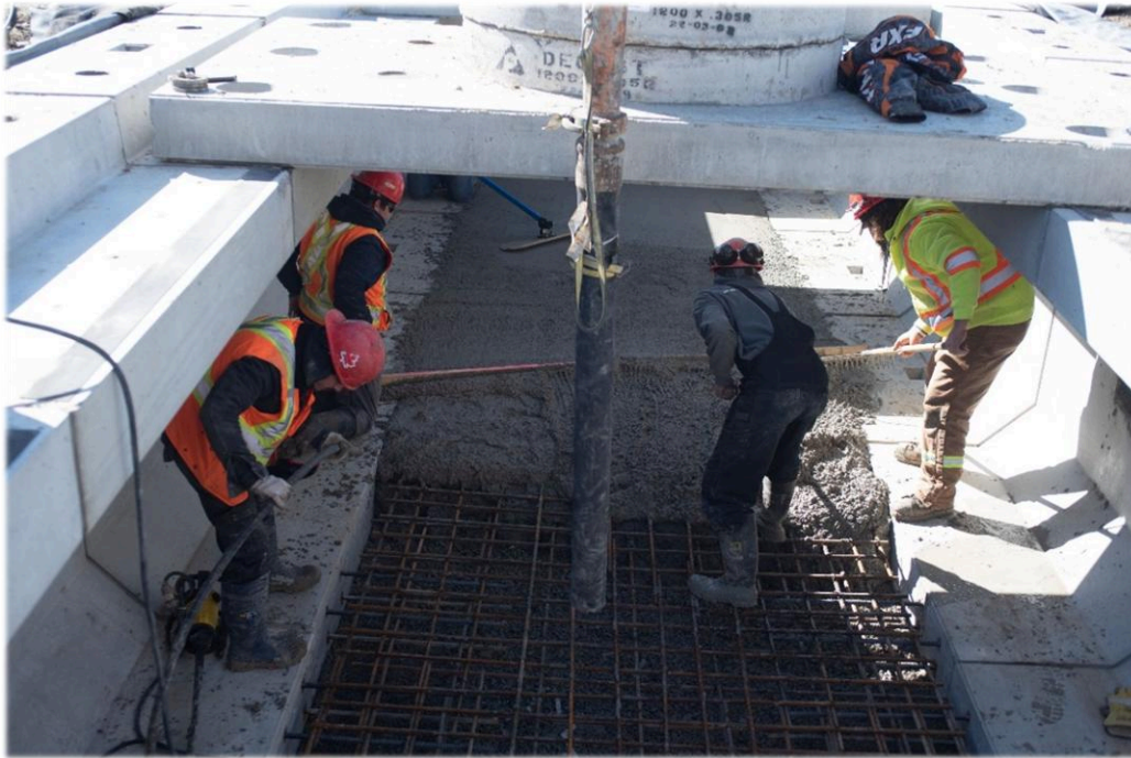
Figure 24: Pumping concrete for cast-in-place floor
