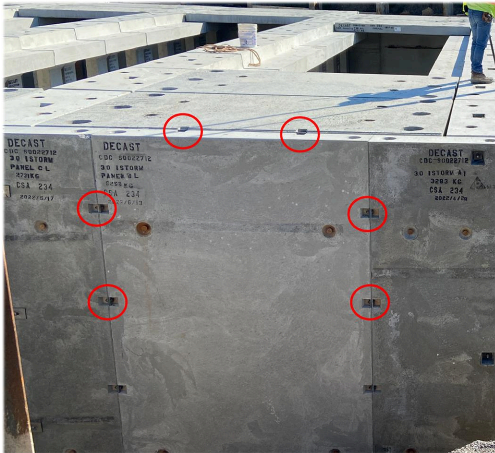
Figure 20: Bolted panel connections on site
