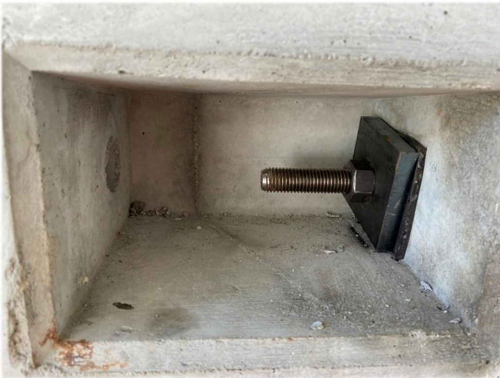
Figure 15: Connection hardware configuration - site example
