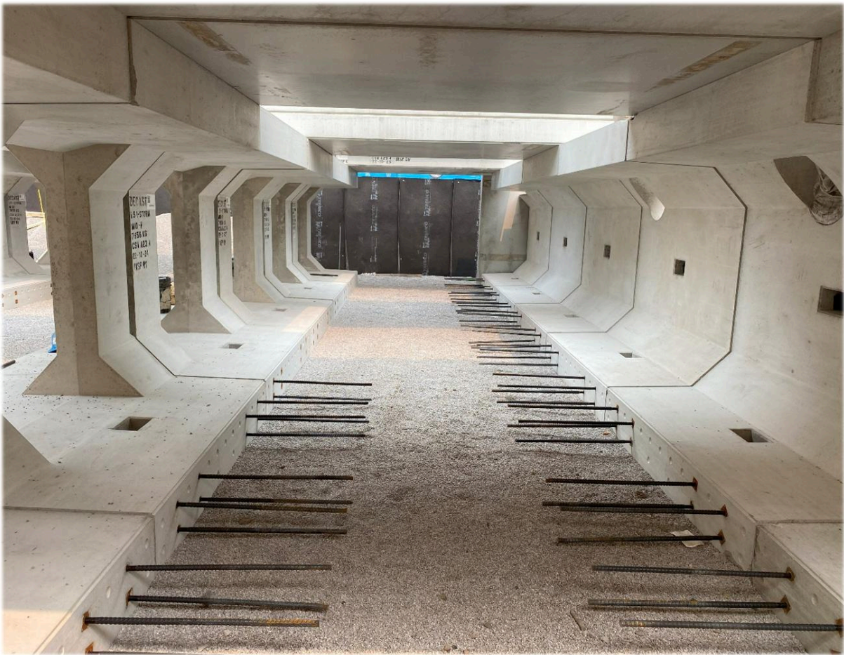
Figure 21: Dowel inserts in tank floor
