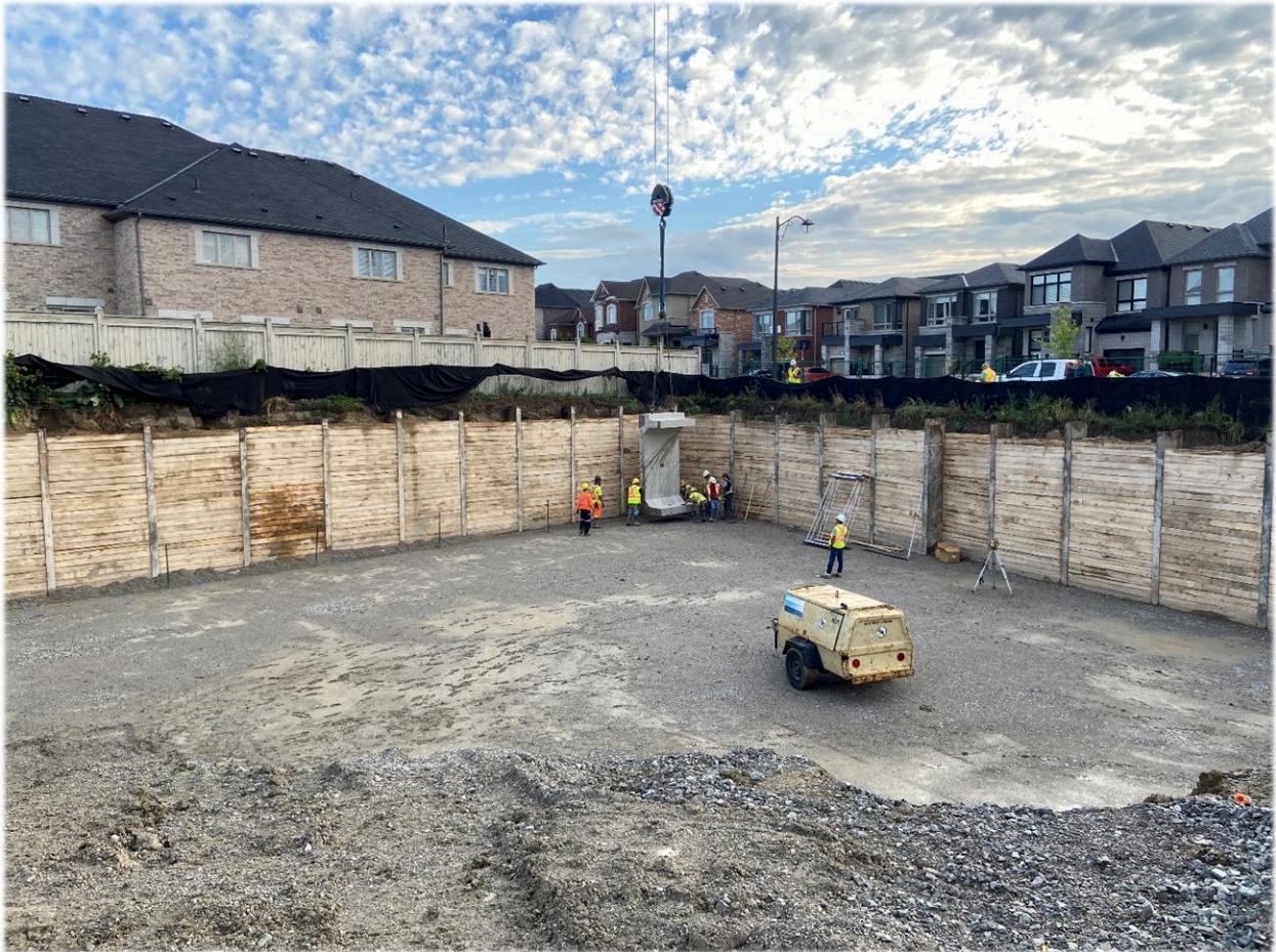
Figure 12: Installing first end unit
