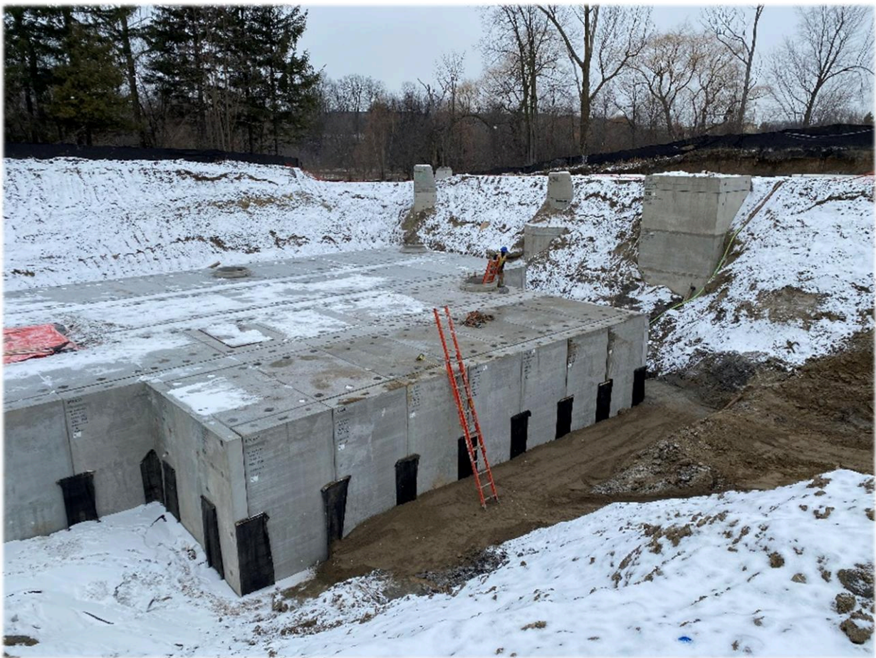
Figure 28: Backfilling around the tank
