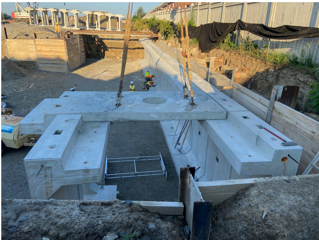
Figure 9: Installation Sequence 4 - Corner top slabs
